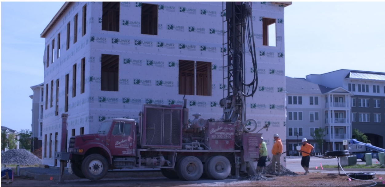
Live drilling project onsite April 2023
