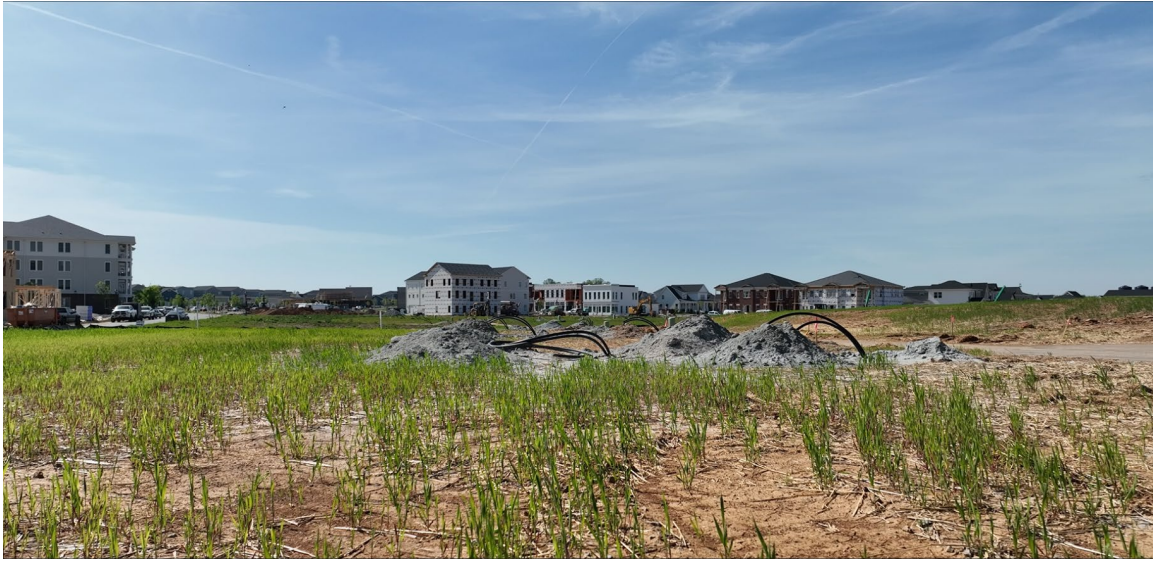
Loop installation prior to construction April 2023
